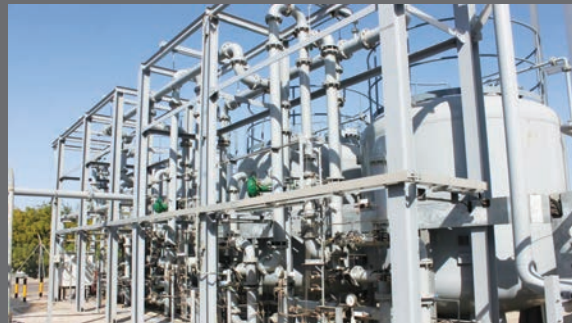
MB - ACF Plant in Oman
